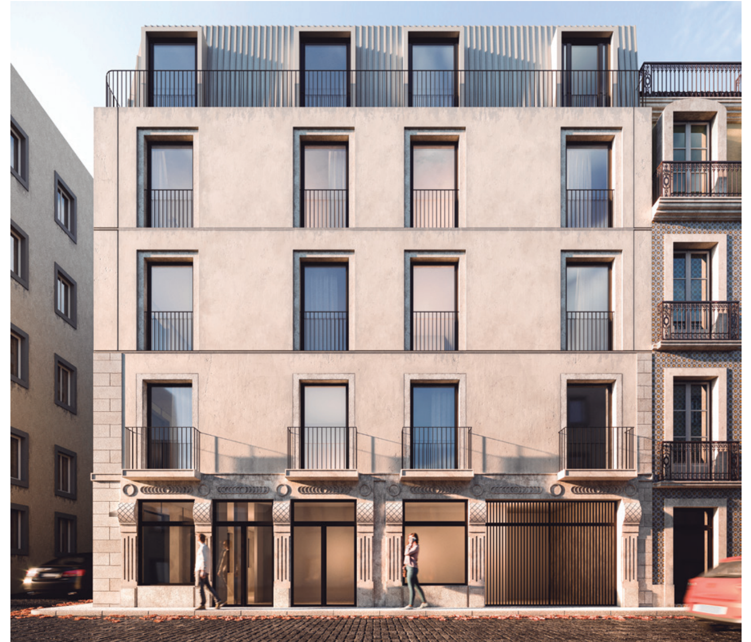
Main Facade, Block A Fachada Principal, Bloco A
